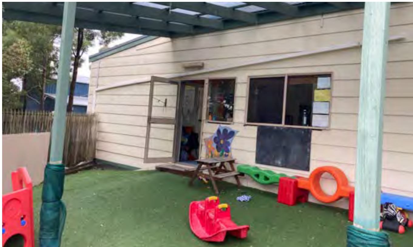
At north ground line locally mounded to provide access to children's rooms
