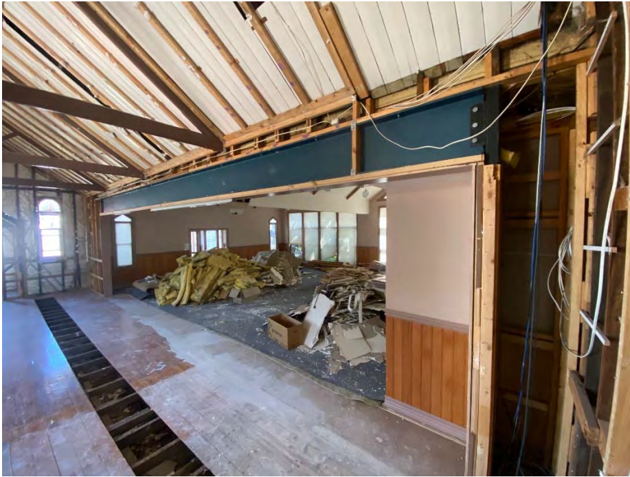
Interior, former Church, undergoing dismantling showing large introduced opening in the longitudinal elevation, February 2020. This elevation was reconstructed.
