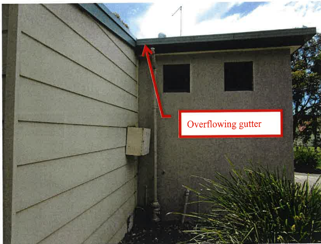
Photo 3; Building south east re-entrant corner.
