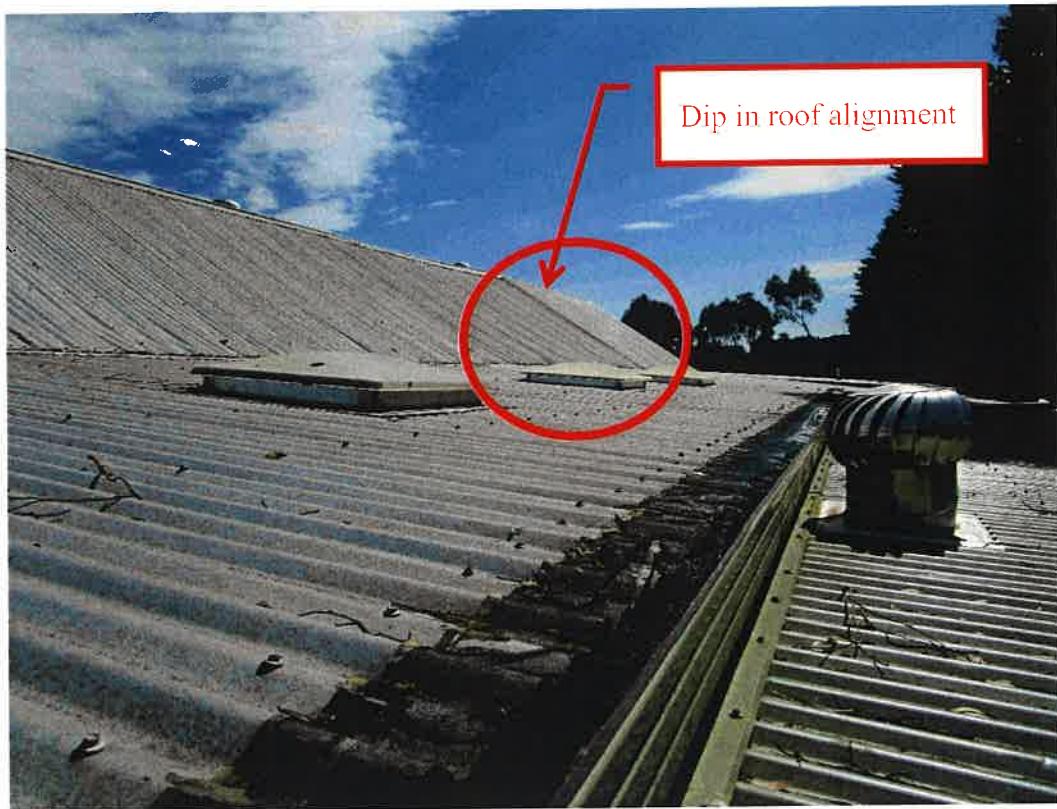
Photo 9; North side of roof
