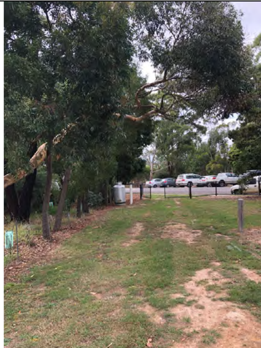
Figure 16- LP Gas tank located in NE corner of site
