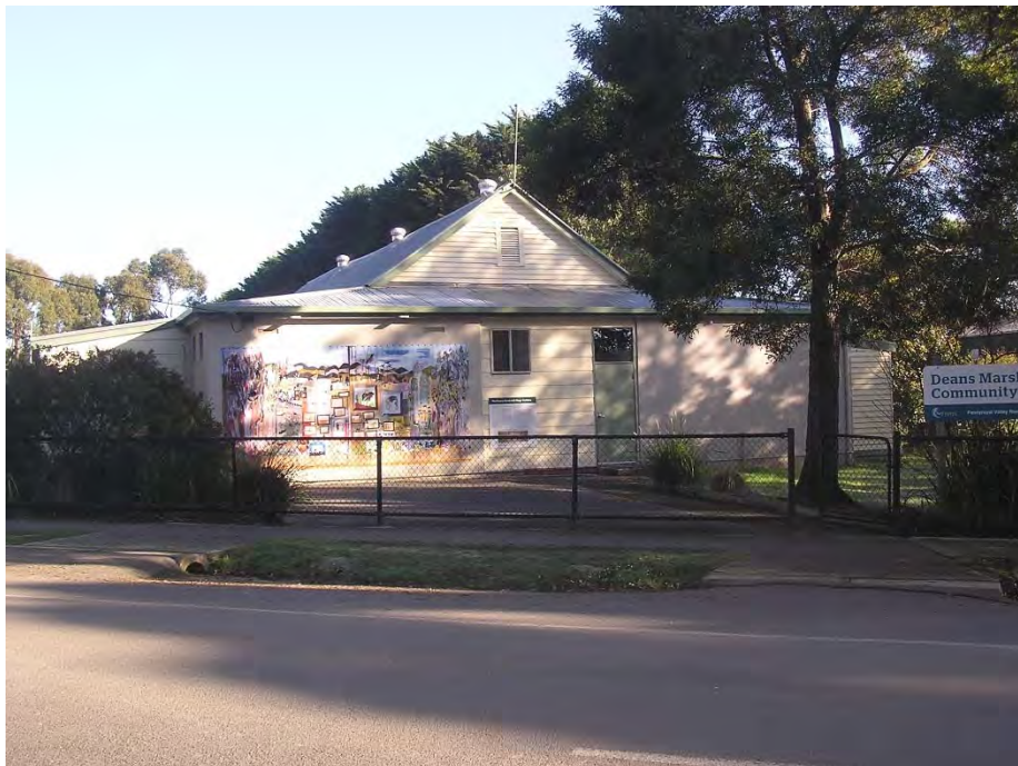
Deans Marsh Hall, east elevation showing early gable end with ventilator, July 2022.
