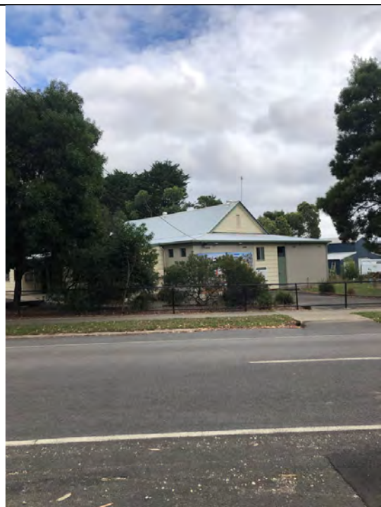
Figure 5- Existing overhead supply to the Hall from Pennyroyal Valley Road
