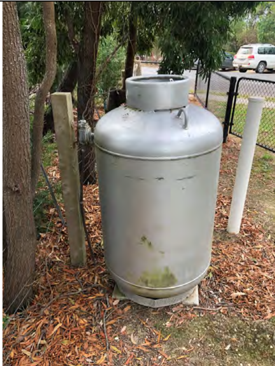
Figure 15- Onsite LP gas storage tank
