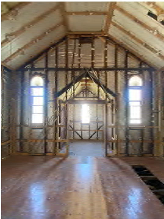
Interior, former Church, undergoing dismantling, February 2020.
