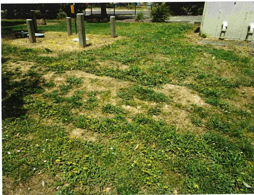
Photo 5; Septic tank location, within bollards. Uneven soil surface allowing for water ponding.
