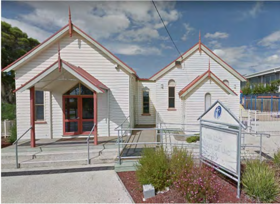
Former Church (right) and introduced hall (left), fronting Balmoral Crescent, Rippleside, prior to dismantling, relocation, reconstruction and adaptation, March 2015. Source: © Google Streetview.
