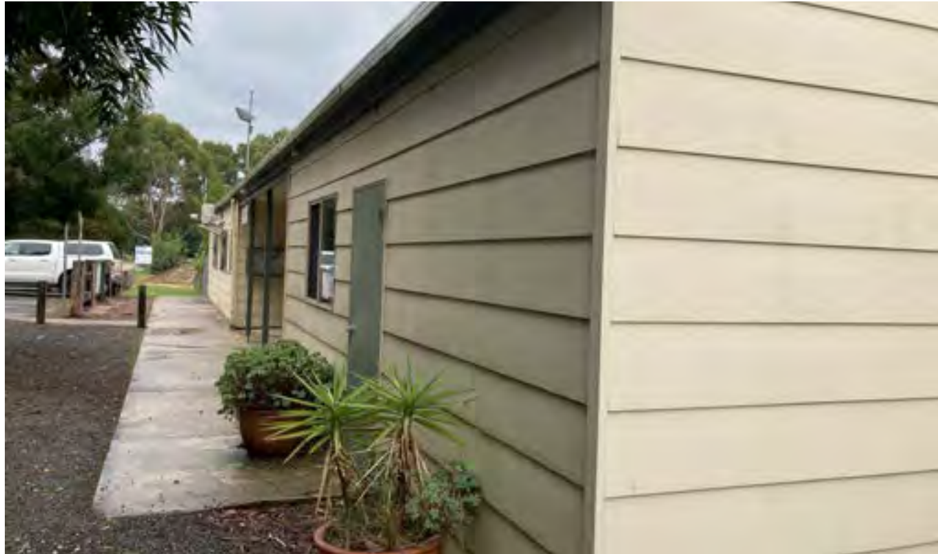
Western facade floor at ground level with combination of pavement finishes
