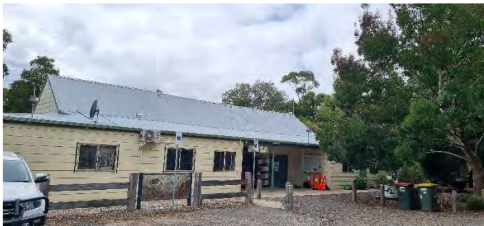
Site conditions – Photo from the carpark showing the community hub building to the north
