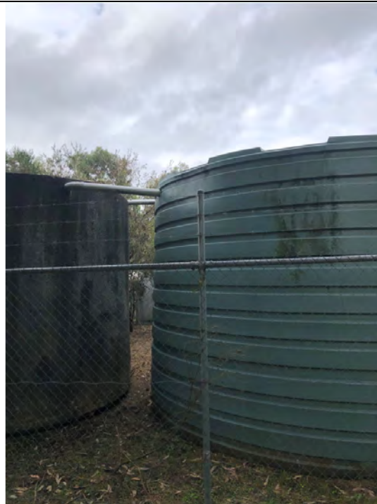
Figure 14- Rainwater tanks of varying age, type and condition located in tank farm
