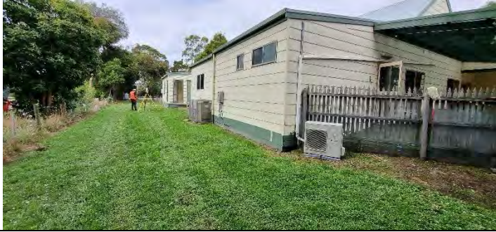
Site conditions – Facing east, photo along the north face of the community building
