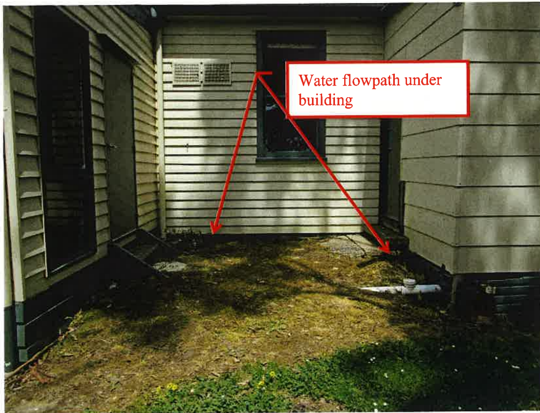
Photo 7; North courtyard; soil surface level higher than under building.
