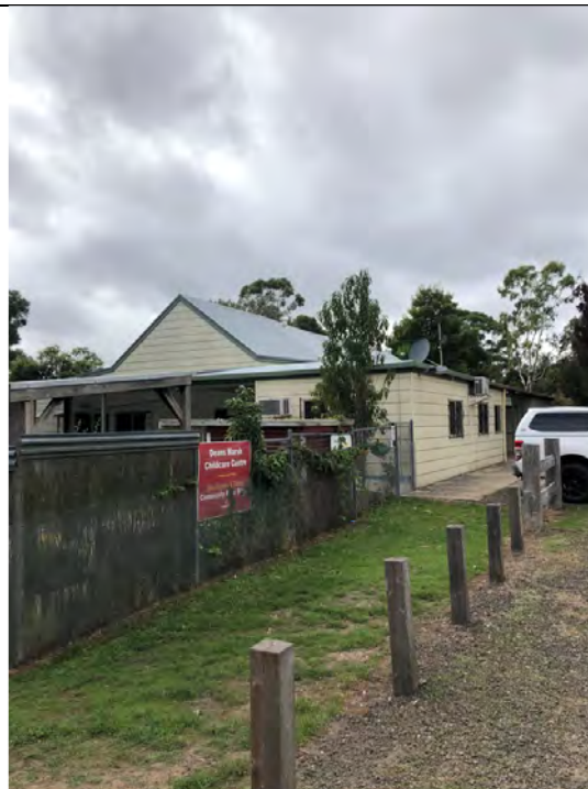
Figure 26- NBNC fixed wireless receiver located at roof level
