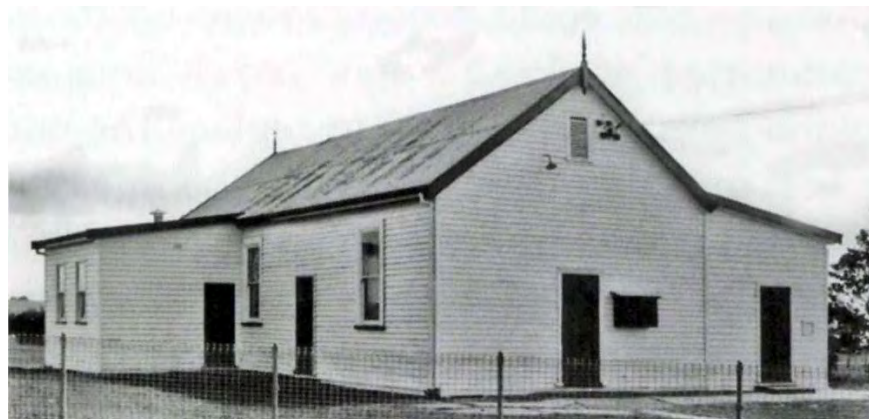
Deans Marsh Hall, east & south elevations showing skillion-roofed supper room addition, c.1960. Source: P. Baragwanath & K. James, These Walls Speak Volumes: A History of Mechanics' Institutes in Victoria , Pam Baragwanath & Ken James, 2015, p.183.
