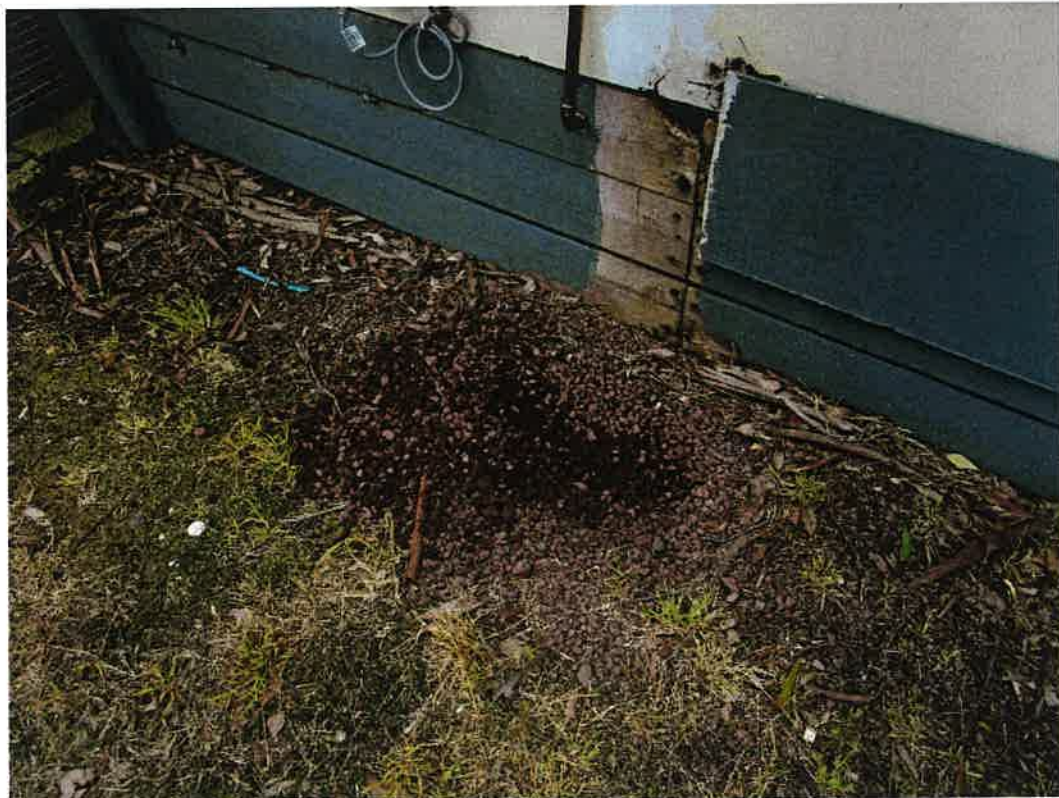
Photo 8; North side. Scoria filled hole. Purpose unknown.
