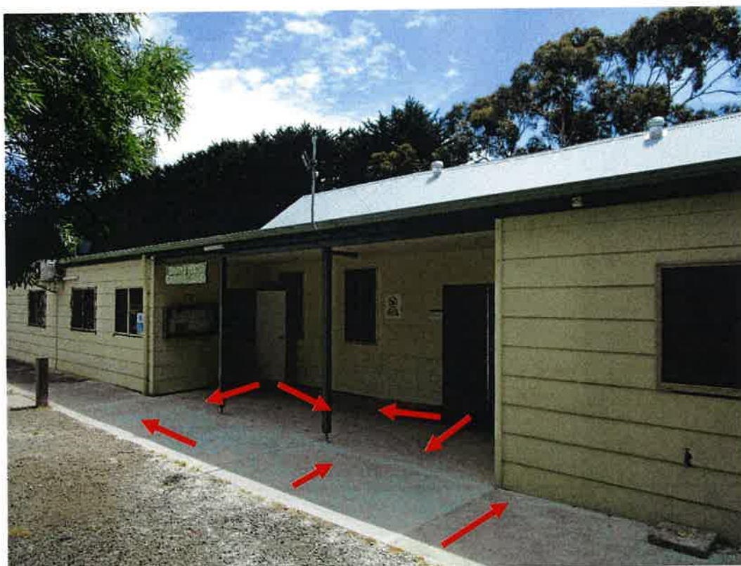
Photo 2; South of hall. Arrows show direction of paving fall.
