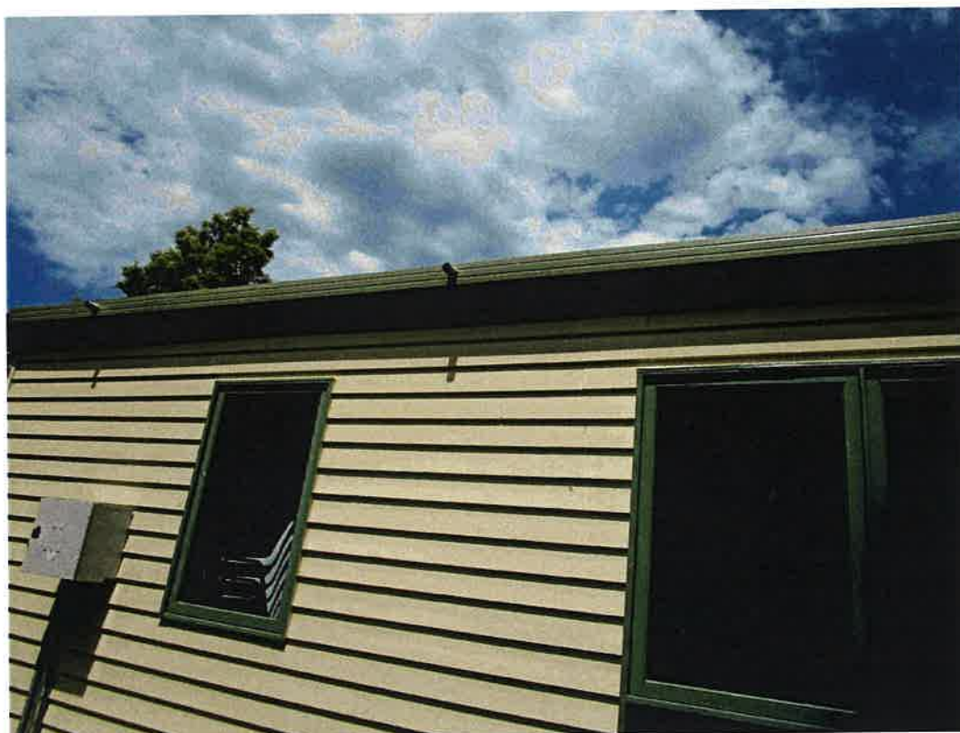
Photo 6; North gutter showing overflow outlets.
