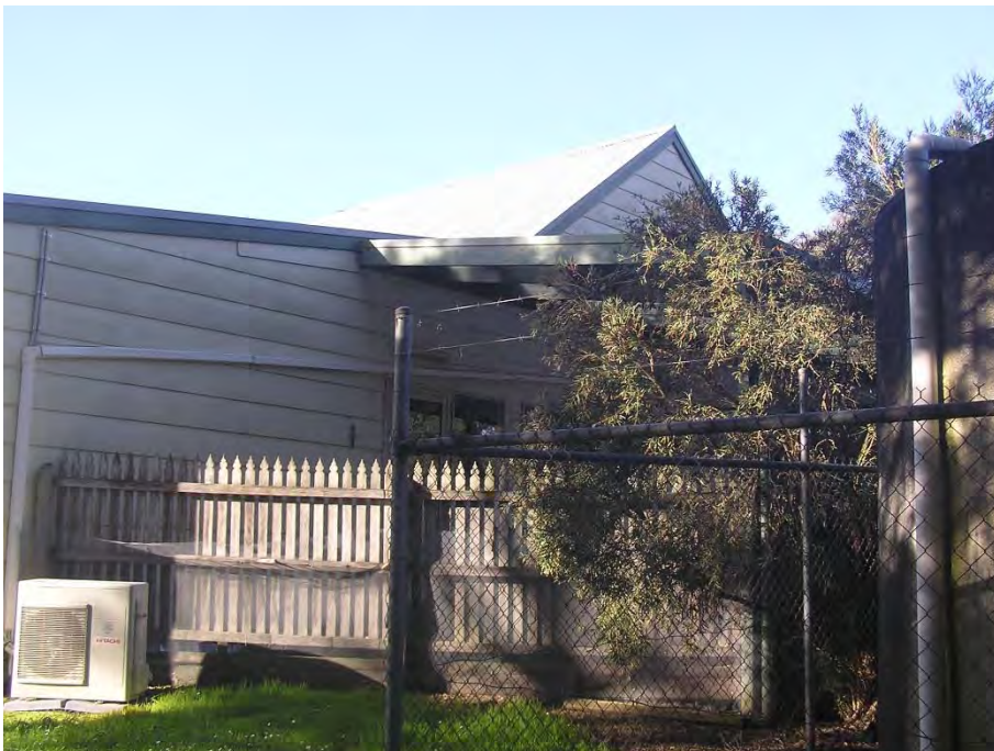
Deans Marsh Hall, west elevation showing additions of 2000, July 2022.
