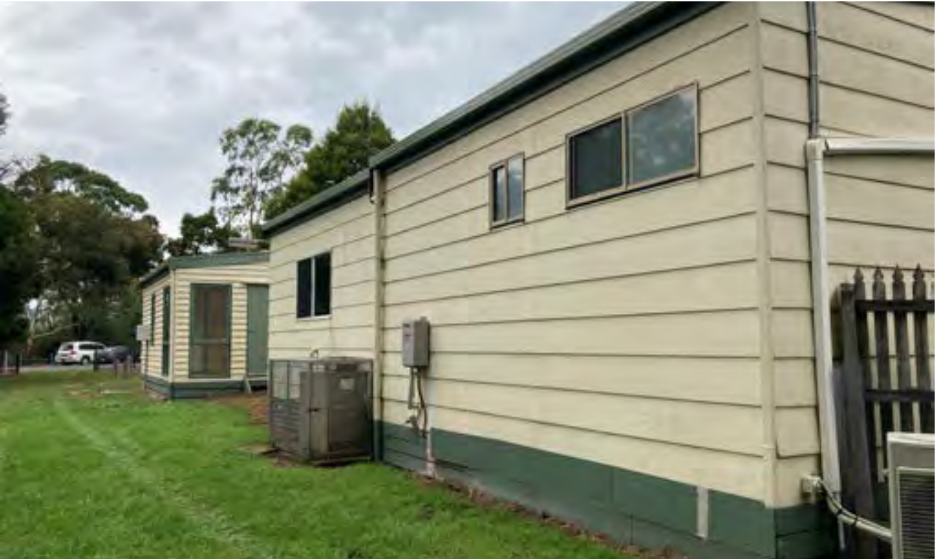
Eastern facade floor approx 400 out of ground mixed lightweight cladding
