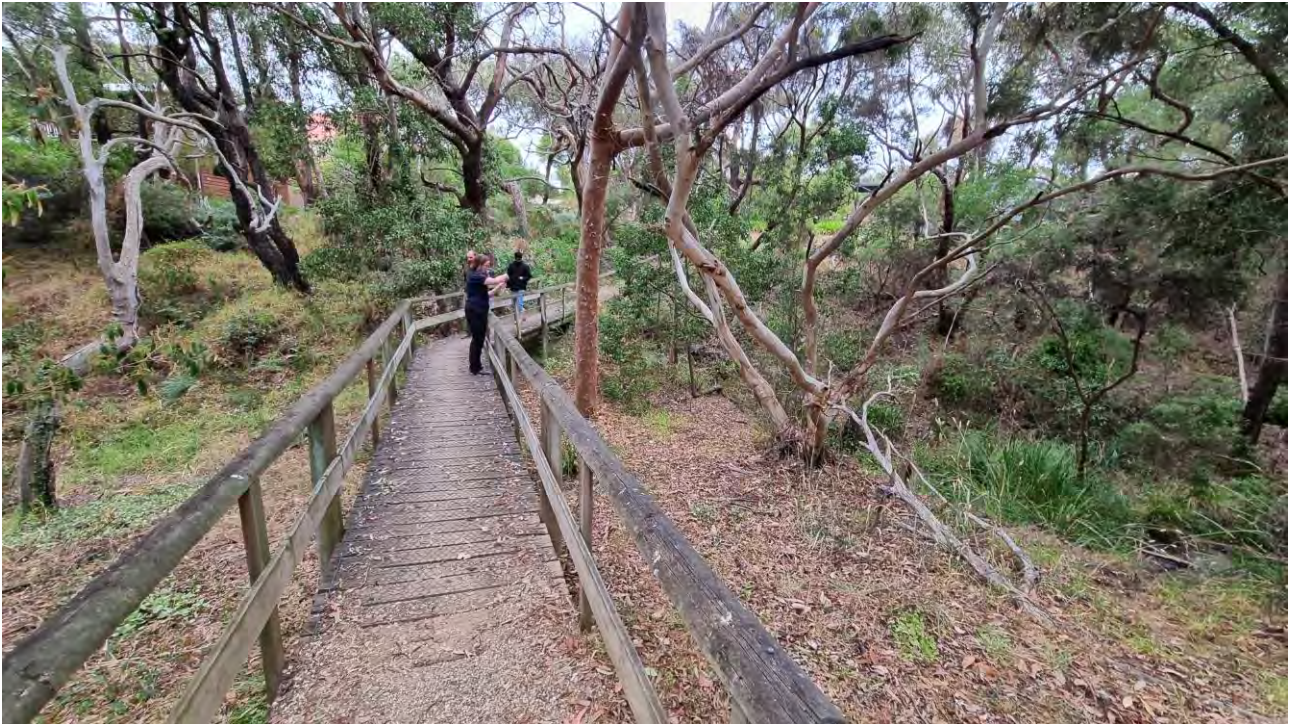
Figure 2-7 Aireys Street Pedestrian Foot Bridge – Facing West
